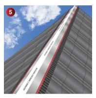
Roll out the ridge roll centrally across the entire length of the ridge batten, using the white spine of the roll as a guide over the ridge batten. Secure the roll by nailing or stapling through the white spine. All joints in the ridge roll must be overlapped by 75mm min. Leave a 75mm long strip of the roll at each end of the ridge.
