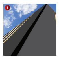
Install the underlay and battens as normal, leaving the underlay 5-30mm short of the ridge on both sides. Do not fix the top tiling batten at this stage.
