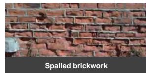
Spalled brickwork
